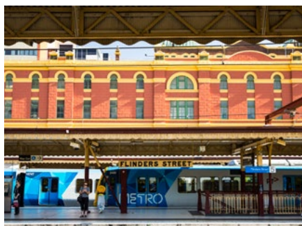
Above: Flinders Street Station
